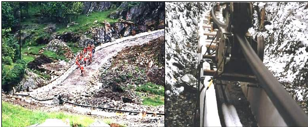
Figure 40 – Submarine cable installation (land operations)
