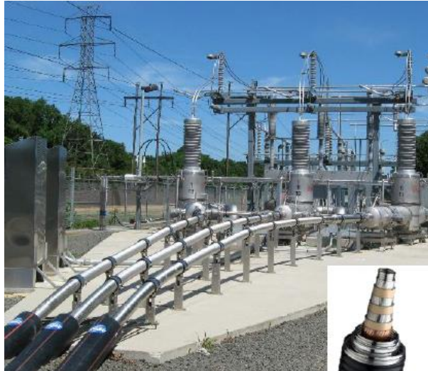
Figure 35 – HTS Installation
